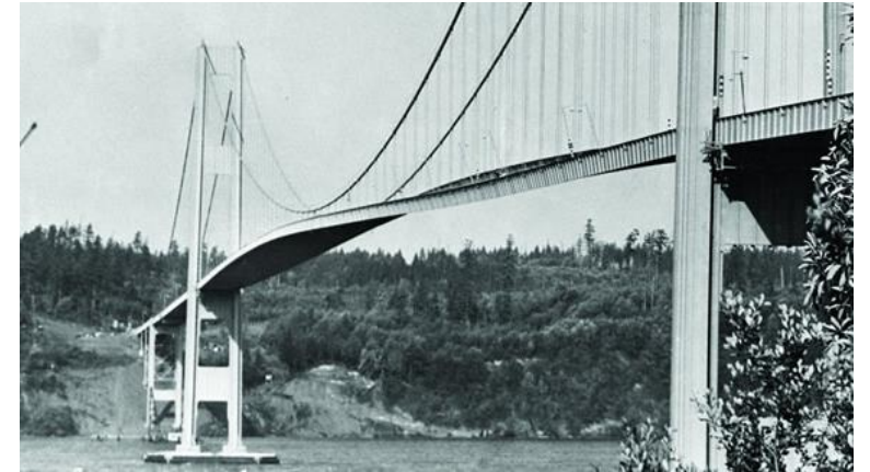
Tacoma Narrows Bridge opened in July 1940, but collapsed due to aero-elastic flutter four months later.
